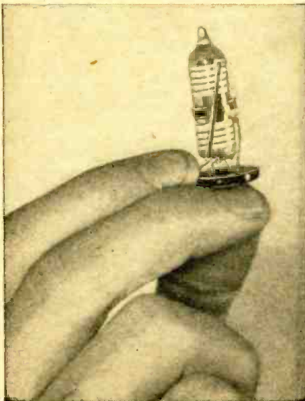
"Lipstick" transmitter used by Dr. Brunetti.
