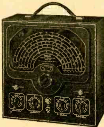
Fig. 3—Substitution box for r.f. capacities.
