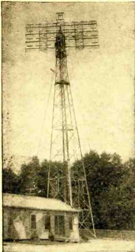
Photo C—High-elevation 32-element billboard.
